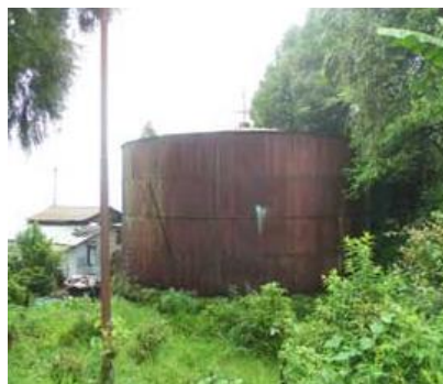
Figure 4. St. Paul Water Tank
