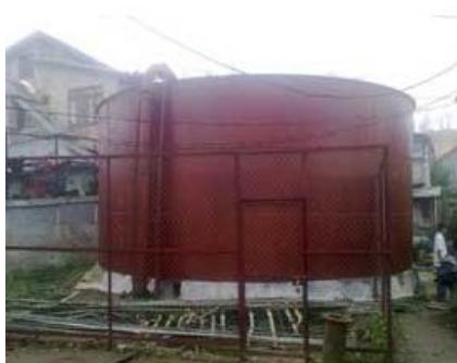
Figure 3. Rockville Water Tank
