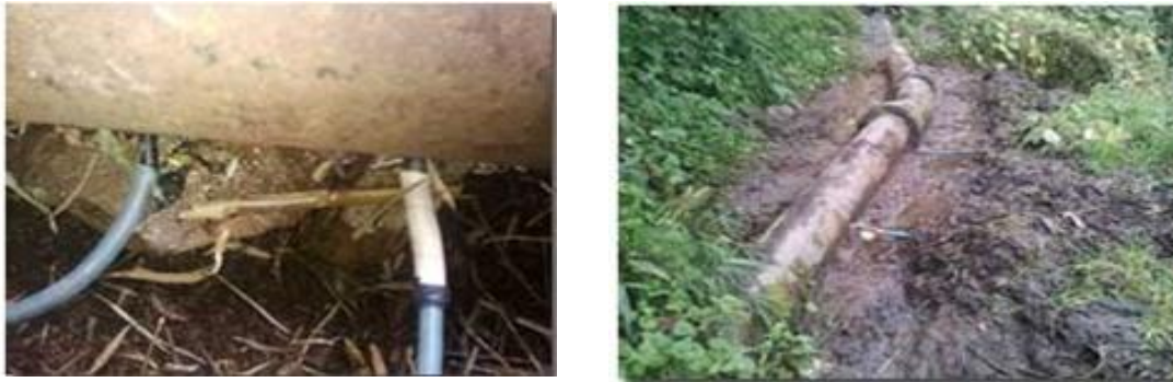
Figure 11. Illegal tapping of water in the main transmission line at Aloobari, Ganeshgram
