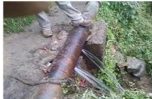
Figure 10. Illegal tapplings of water in the main transmission line at Rangbull & Aloobari, Ganeshgram
