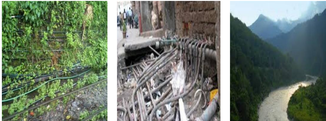
Figure 16. Water supply in Darjeeling (Bindu Dam)
